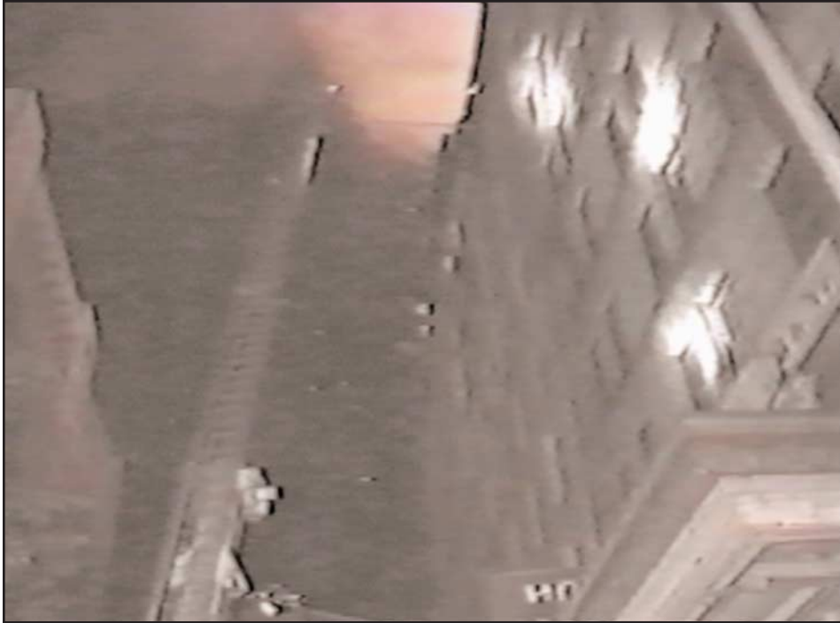
3. Conditions from the street.
