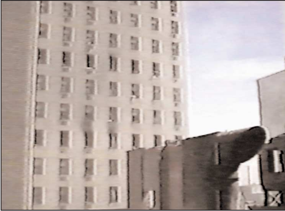
10. Damage to exposures across Clark Street from the fire building.
