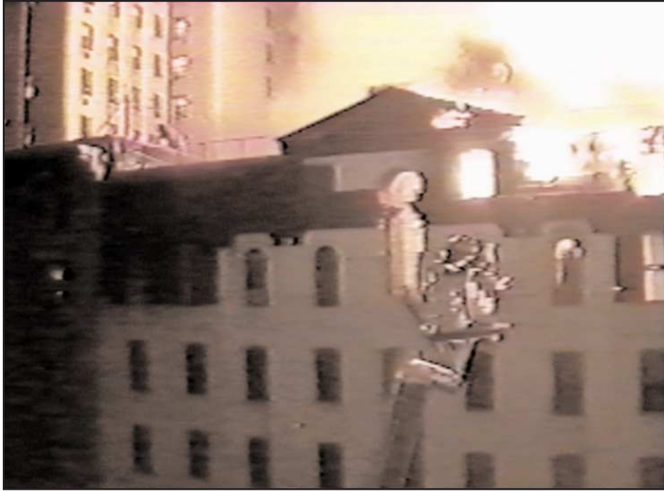
1. Early conditions on the Clark Street (front) side of the Clark building with Truck 119 in position to operate its elevated master stream.
